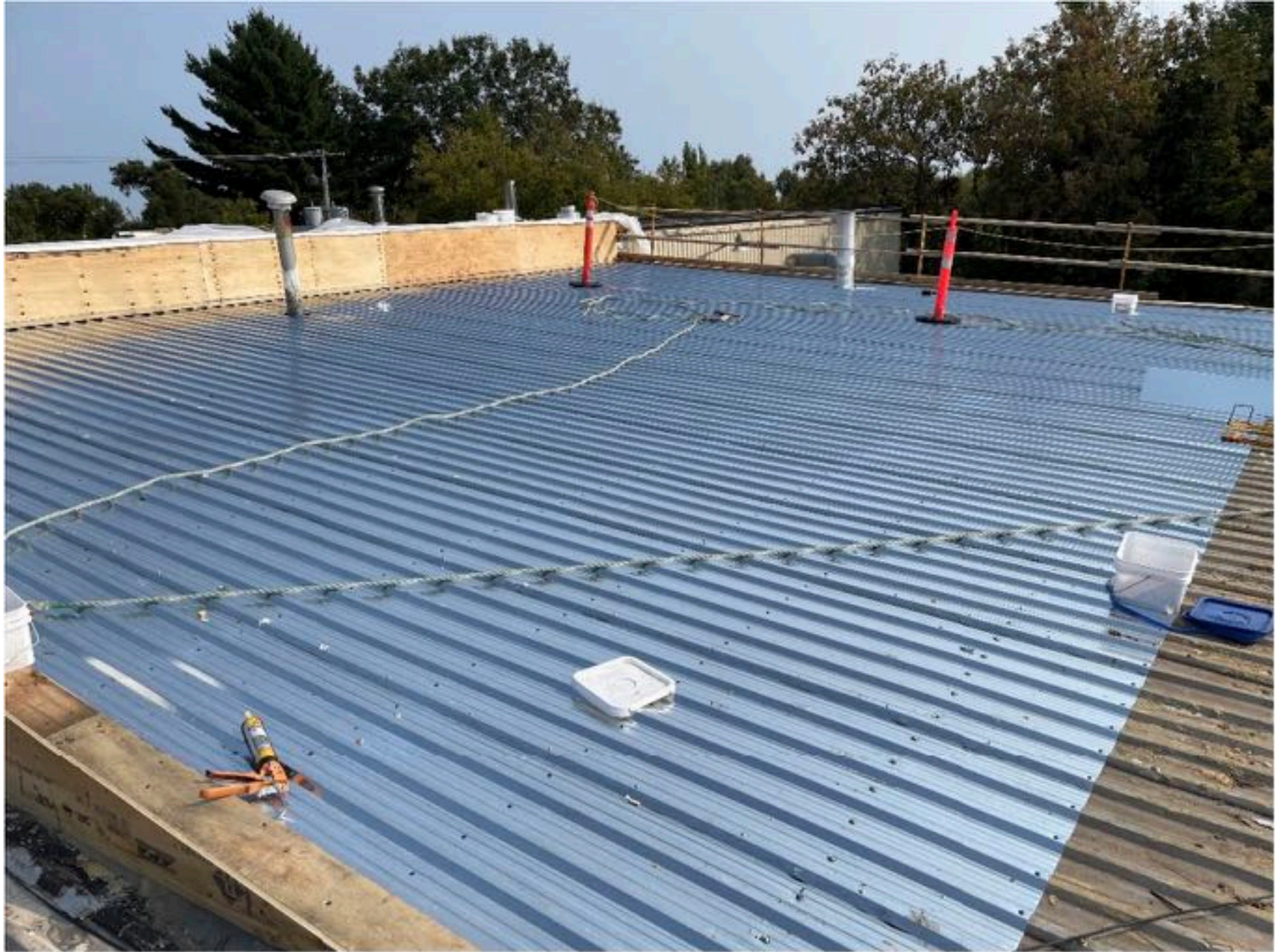
5.2 New Roof Panel Installation Complete
