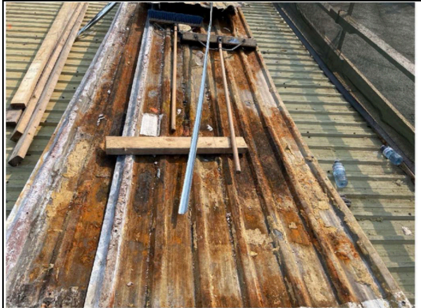
5.3 Typical Condition of Existing Roof Panels that were Replaced
